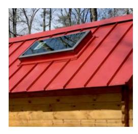
**Design:** Hidden fasteners, interlocking panels (12"-18" widths), custom cut or pro-installed.
